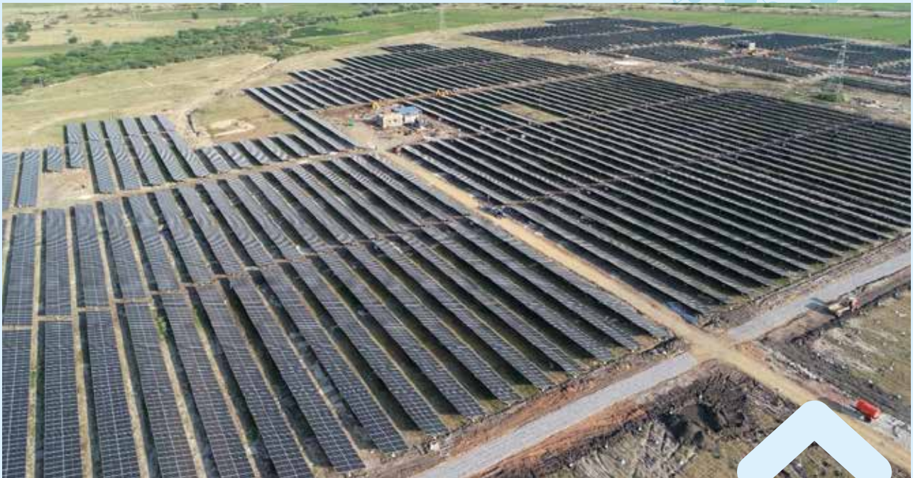
14 MW captive solar power plant at Raichur, North Karnataka, that helps us to meet our 'green energy' goals
